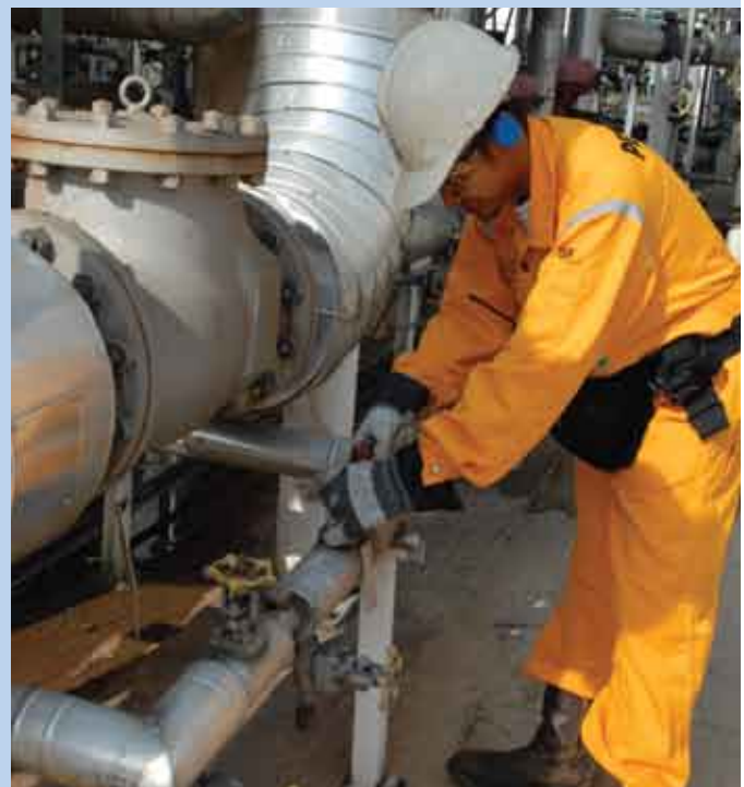
Maintenance work on a steam trap at PP(M)SB
