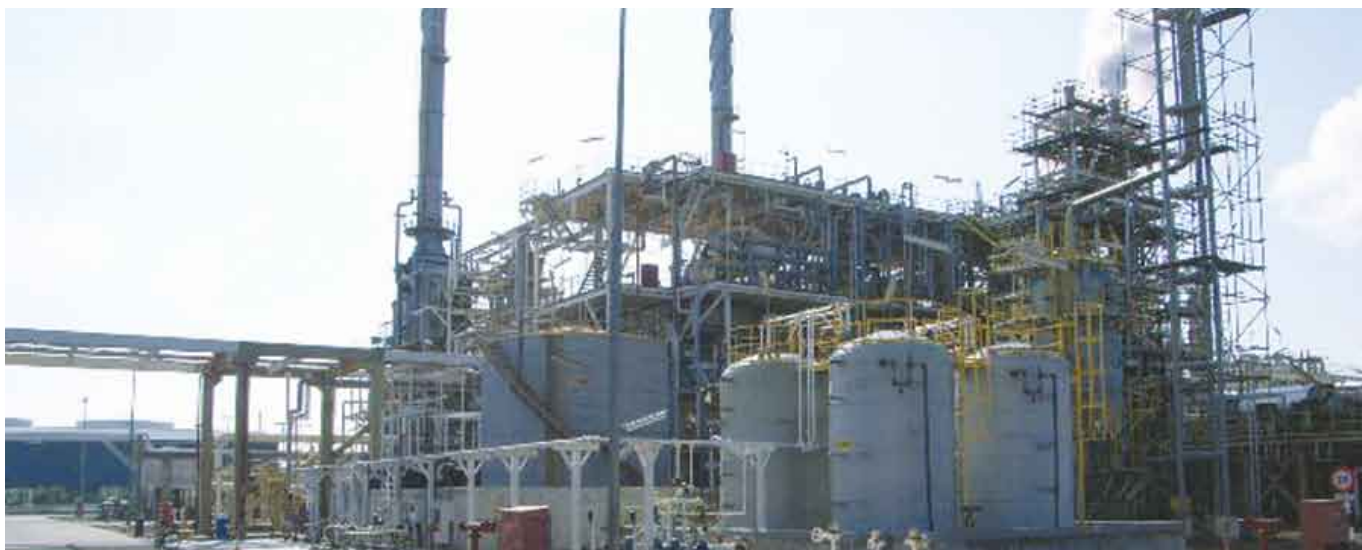
The 33 per cent HCl Project storage and pump facility (in the foreground) at VCM
